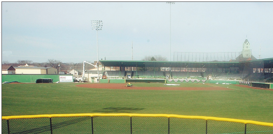
Alliant Energy Field has been under construction due to renovation funds provided through the Vision Iowa program.
